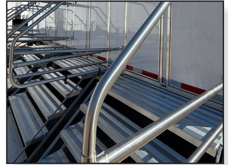
Flip-down steel step assemblies with lighting.
