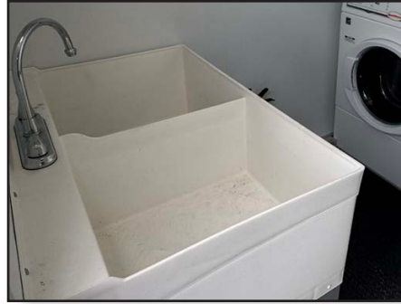
Two-bay utility sink
