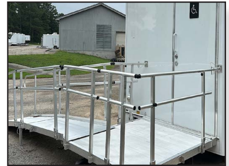
Accessible ramp meets ADA requirements.
