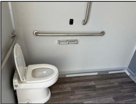
Accessible grab bars assist with sitting, standing and transfers.
